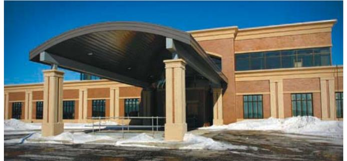
building's walls are made of recyclable and energy-efficient precast concrete. Such material is often made in a nearby region, which is considered environmentally friendly because less fuel is used for delivering materials. In this case, the precast concrete was made at Wells Concrete in Albany. Its high-insulation roof is also made of a precast plank.
