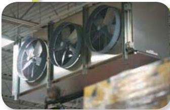
**WASHING TRUCKS:** C&L's trucks need to be washed about once a week. So it takes the heat generated from its cooling system and uses it to warm the 100-gallon water tank used to wash its vehicles. The system cost about \$4,000-\$5,000.
